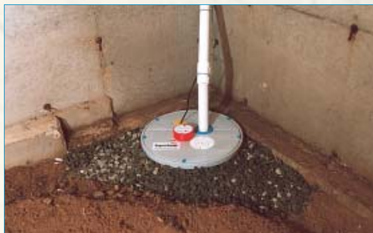
The SuperSump™ will be installed in a low spot in your crawl space. As an option, a drainage swale or trench system can be developed around the perimeter to drain water to the SuperSump™. An UltraSump™ battery back-up pumping system is an option.
