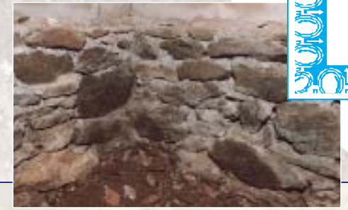
Walls made of block or stone often let moisture into a crawl space. That's why it's important for a solution to include the walls as well as the floor.
